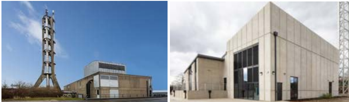
Figure 2. Campus West and East Energy Centres
